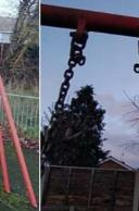
Action: Monitor for any further deterioration and replace Finding: There is some wear to the shackles when 40% worn
