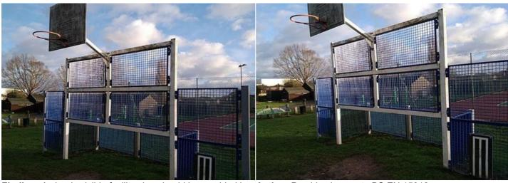
Finding: A clearly visible facility sign should be provided in Action: Provide signage to BS EN 15312 a prominent position with the wording as detailed BS EN 15312- the equipment is not intended for children less than 3 years old- the warning - Do not climb on the framework or nets- the warning - Do not hang on the ring (if provided)- the warning - Do not wear rings or other jewellery- name and telephone number of the administrator- number to call in case of accident
