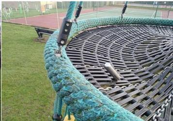
**Finding:** There is/are finger entrapment/s in the basket slots **Action:** Monitor - No remedial work recommended and the item fails to meet the requirements of BS EN 1176
