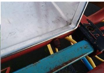
Action: Replace all corroded fixings
