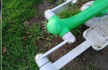
**Finding:** There are gaps between 8 and 60mm creating a potential crush/shear point in contravention of the requirements of BS EN 16630
