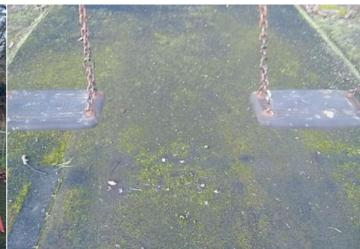
Finding: The safety surface around the area is beginning to Action: Monitor for any further deterioration and repair as required wear
